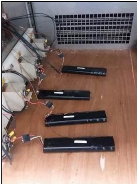
Photograph 13: External Short Circuit Test Setup, SN 09-12
