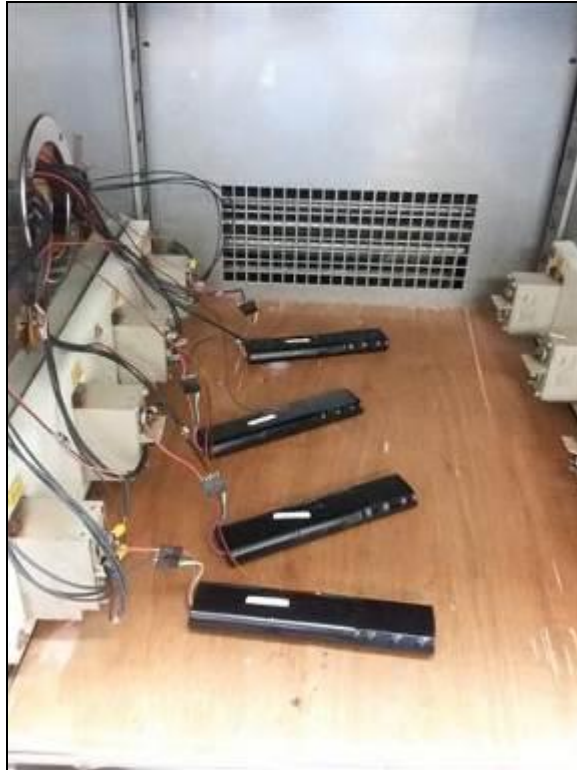
Photograph 12: External Short Circuit Test Setup, SN 01-04
